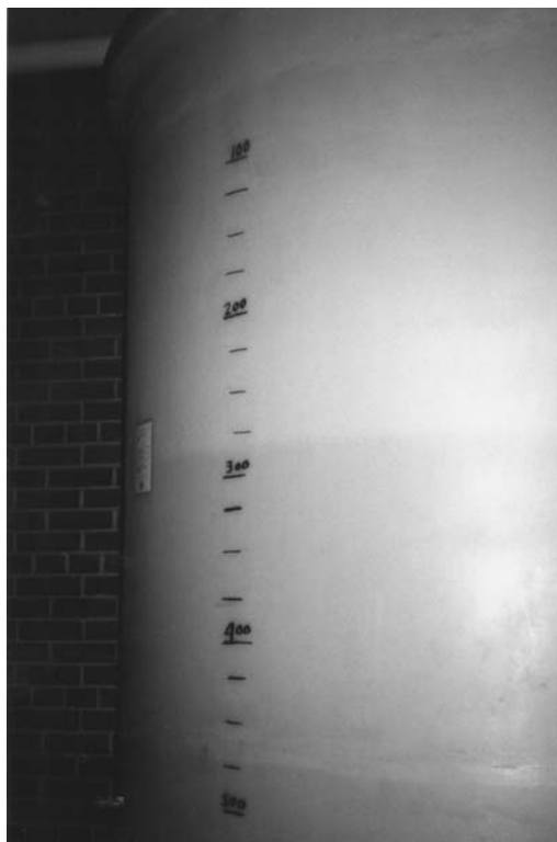
Figure 36.6 Sight gage scribed on polyethylene chlorine contact tank, Cornwall Sewage Treatment Plant, Cornwall, Ont.
