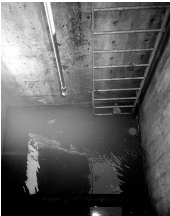
Figure 36.14 Ultrasonic sensor mounting in a sewage wet well, Iroquois Sewage Treatment Plant, Iroquois, Ont.
