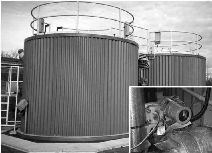
Figure 36.4 Differential pressure transmitter for thermophilic aerobic sludge digesters at the Long Sault Sewage Treatment Plant, Long Sault, Ont.
