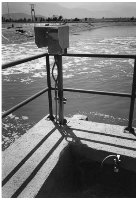
Figure 36.24 Ultrasonic level indicating transmitter on aeration lagoon at the EMOS Wastewater Treatment Plant, Santiago Chile.
