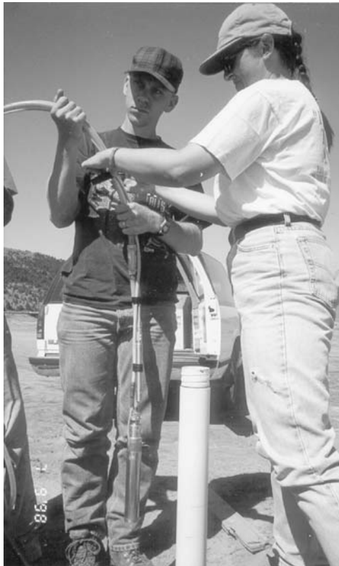
Figure 26.9 Placement of electrician's tape around riser hose and electrical lines.
