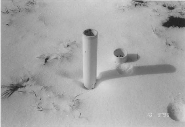
Figure 26.4 Two-inch PVC well with measuring point marked inside the casing.
