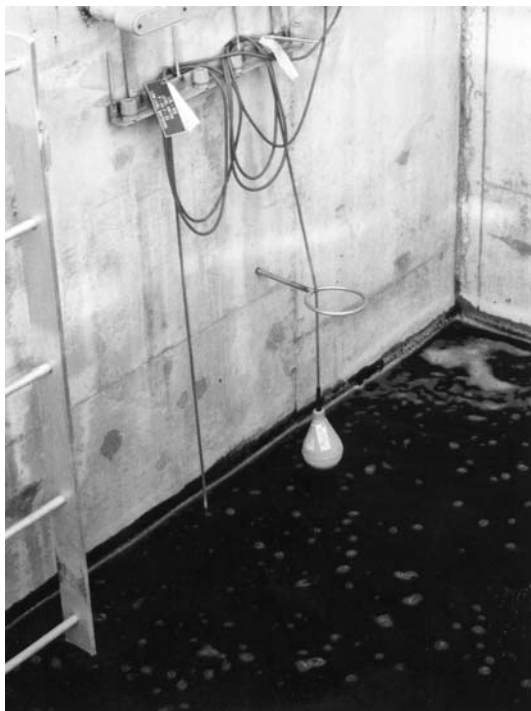
Figure 36.19 Float level control for the effluent contact chamber, Ingleside Sewage Treatment Plant, Ingleside Ont.
