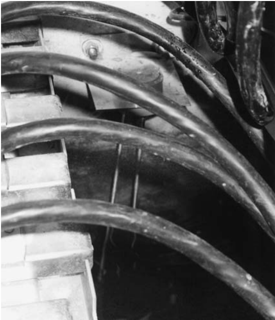
Figure 36.13 Conductance point level control in UV disinfection channel, Long Sault Sewage Treatment Plant, Long Sault, Ont.
