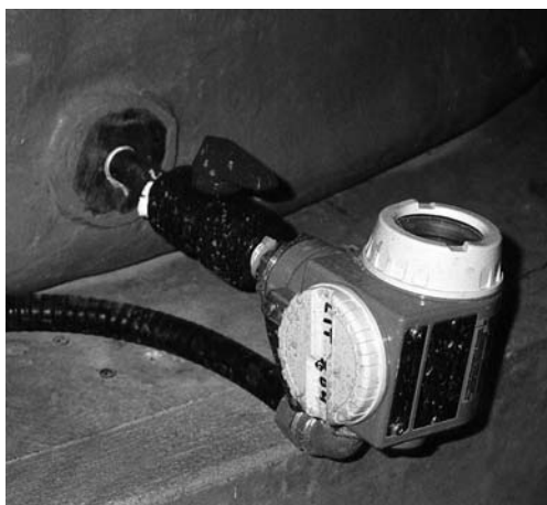
Figure 36.16 Gauge type level indicating pressure transmitter.
