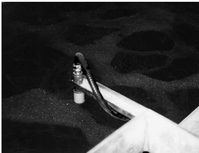
Figure 36.18 Ultrasonic transducer monitoring aeration tank level in the Cardinal sewage treatment plant's sequential batch reactor, Cardinal, Ont.
