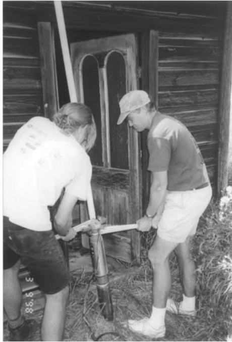
Figure 26.14 Riser pipe and electrical lines extending upward from pump.
