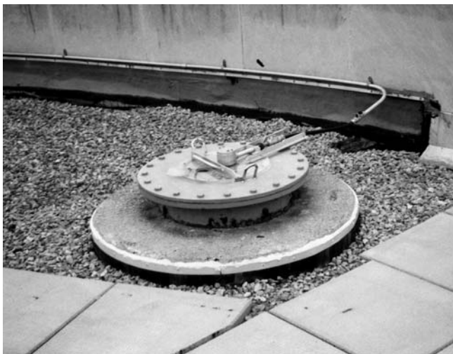
Figure 36.23 Anaerobic digester with ventilated stilling well and ultrasonic transducer, Cornwall Sewage Treatment Plant.
