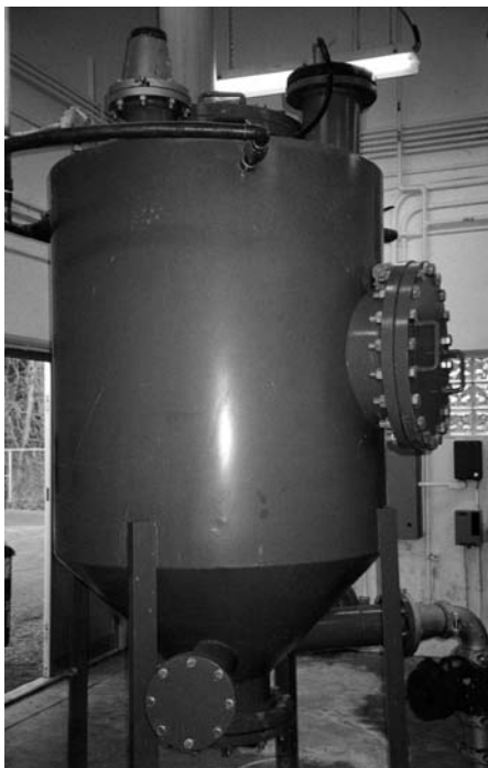
Figure 36.20 Sludge holding tank with ultrasonic level transducer, Ingleside Sewage Treatment Plant.
